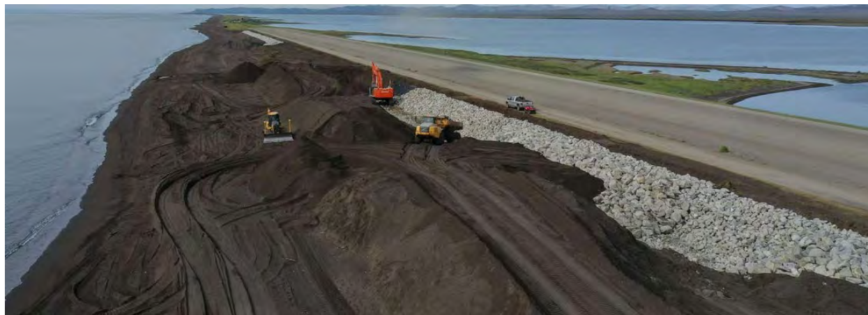
Figure 3. Kivalina airstrip revetment under construction in 2019 (Brice Inc. website)
