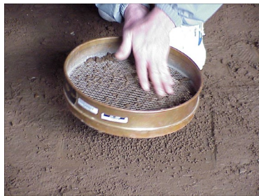
Filling surface voids
