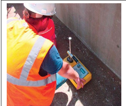
Testing near structure
