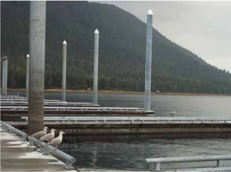
New concrete floating dock in Petersburg, Alaska. The dock rides a short distance up and down the poles, with the tide.
