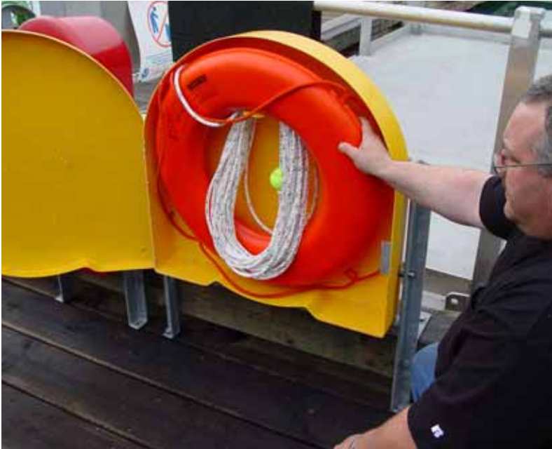
Scott Brown, harbormaster for Dutch Harbor/Unalaska, shows a ring life buoy (RLB) at Valdez Harbor. RLBs should be installed every 75 feet on the floats. Brown uses the same life rings in his harbor.
