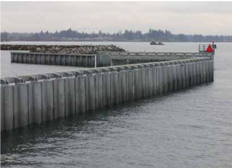
A sheet pile wave barrier forms a vertical barrier to the prevailing waves.
